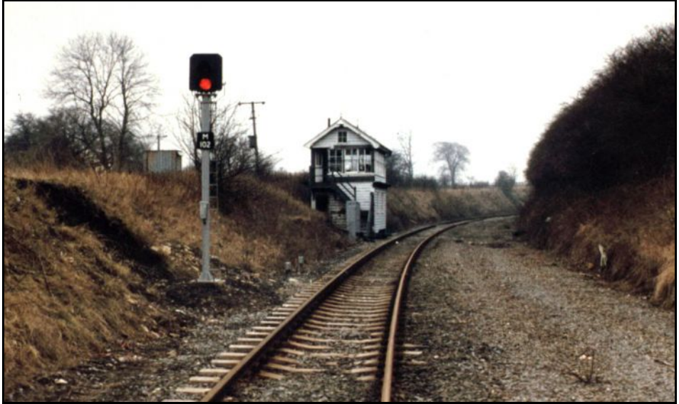
Firbeck "A" signal box viewed from the Doncaster direction. Colour light signal is controlled by Doncaster power box. Evidence of double track formation on the north-west curve is still visible.
