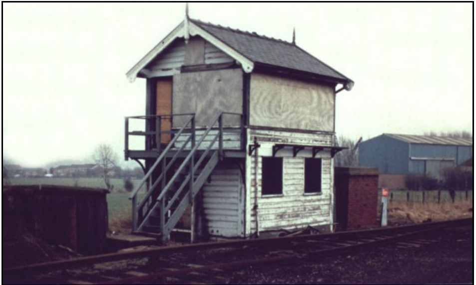
Firbeck "B" signal box with disused north-east curve track in the foreground. Tickhill visible in the background.
